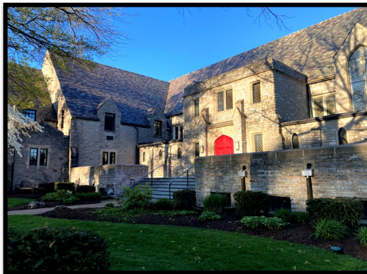
CHPC Member Dick Michaelian recently took this photo of our beautiful church, which has seen its HVAC system upgraded recently and now will be graced with new outdoor signage.
